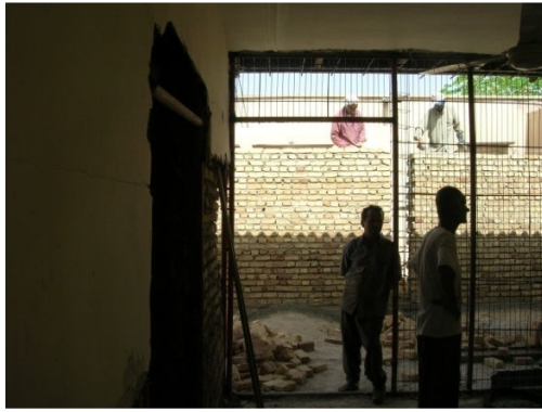
Fig. 18 Workers are demolishing some parts of an original PEH due to heterogeneity of local materials and those applied in original PEHs
