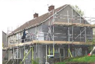
Deep renovation - External wall Insulation
