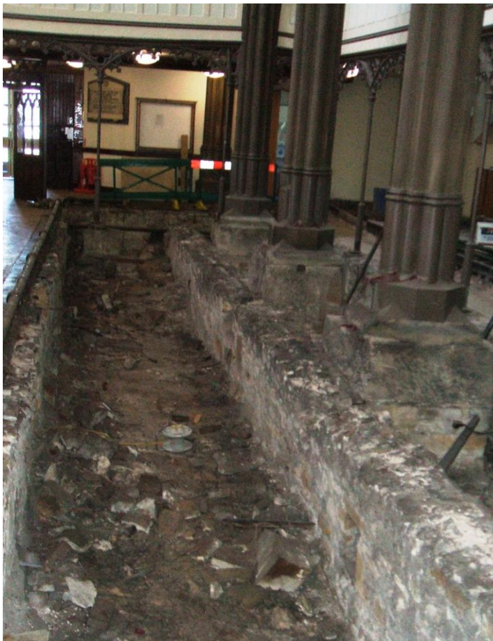
Plate 4.45 Exposed foundations, St George's Chorley, June 2017
