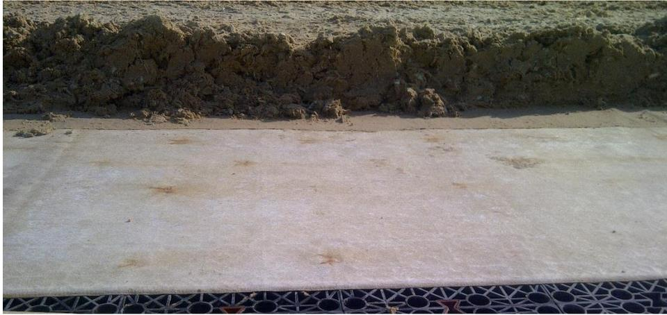
*Plate 5.0.2: Synthetic equestrian surface laid to a depth of 150mm over a Permavoid Limited™ 85 sub-base, separated by a non-woven geotextile membrane.*
