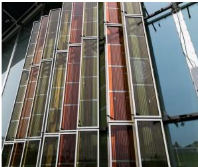
Figure 2.17, Flexible organic solar cells on windows .Adapted from: www.dailyfusion.net/2013/11/swisstech-convention-center-features-multicolored-solar-panel .
