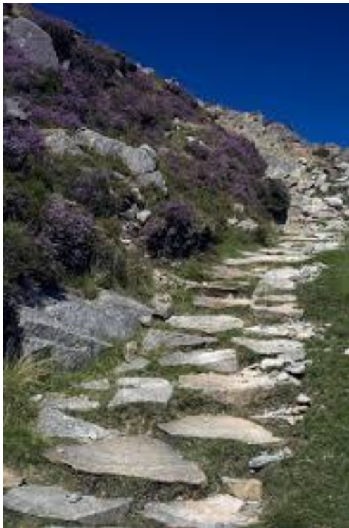
Figure 5.3: Fix the Fells’ step-like structures to combat erosion in the heavily peopled Lake District Fells, available at www.markrichards.info
